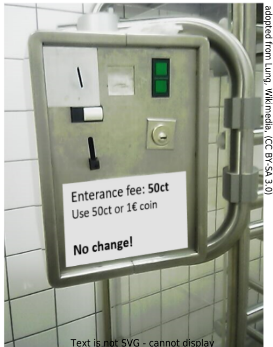
Fig. 11: Entrance Control for Toilets
